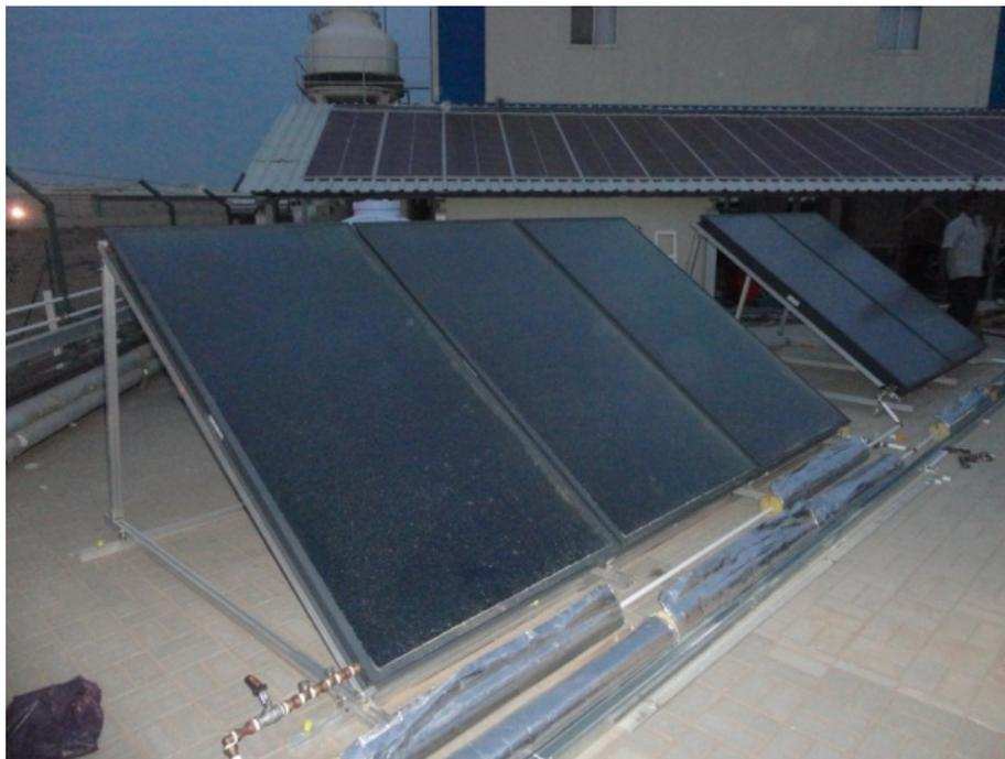
**Fig. 7.** Flat plate collector array aperture area 11.85 m<sup>2</sup> [13].
