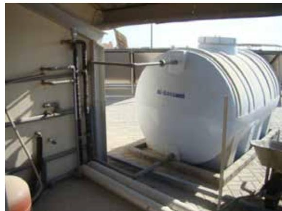
**Fig 4(d).** Cold water storage tank (municipal water supply) [13].
